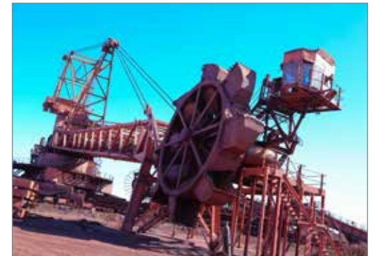
The massive industrial stacker reclaimer at the Saldanha Iron Ore Terminal.
