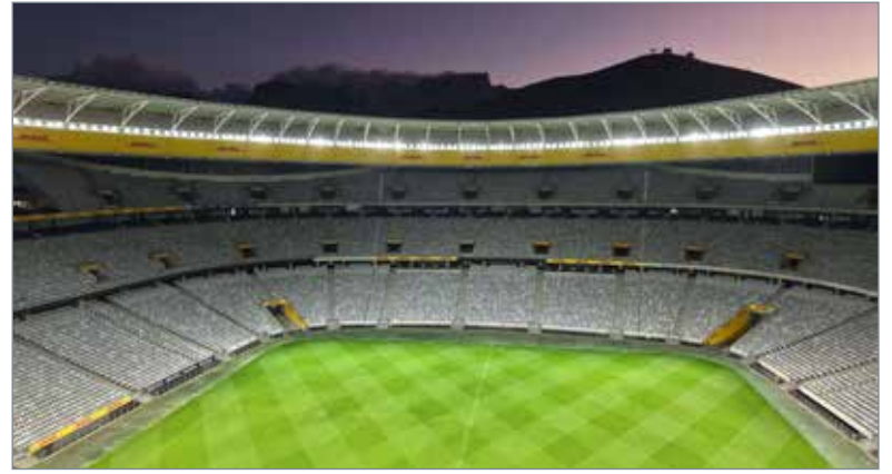
OMNIBLAST floodlights illuminate the DHL Stadium.
