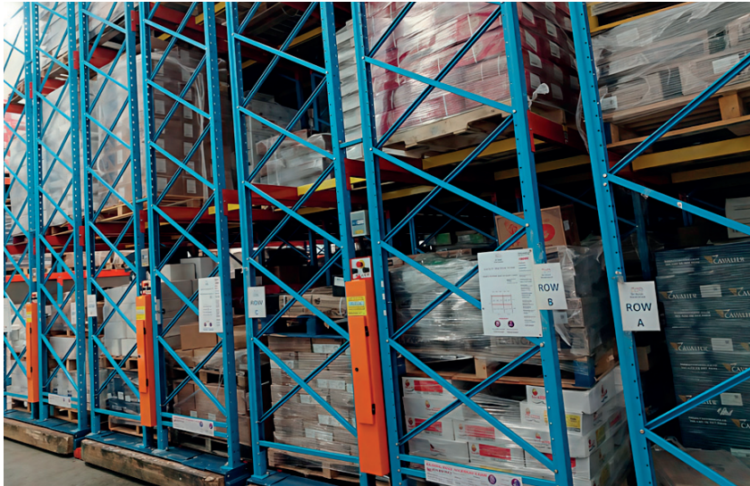
Mobile racking installation within a seafood cold storage facility
