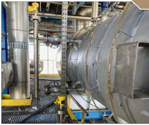
Across three sites, 18 VEGAPULS C 21 80 GHz radar sensors and three VCCS13e cabinets deliver smart, maintenance-free level measurement.
