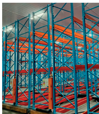
Refurbished mobile base installation
