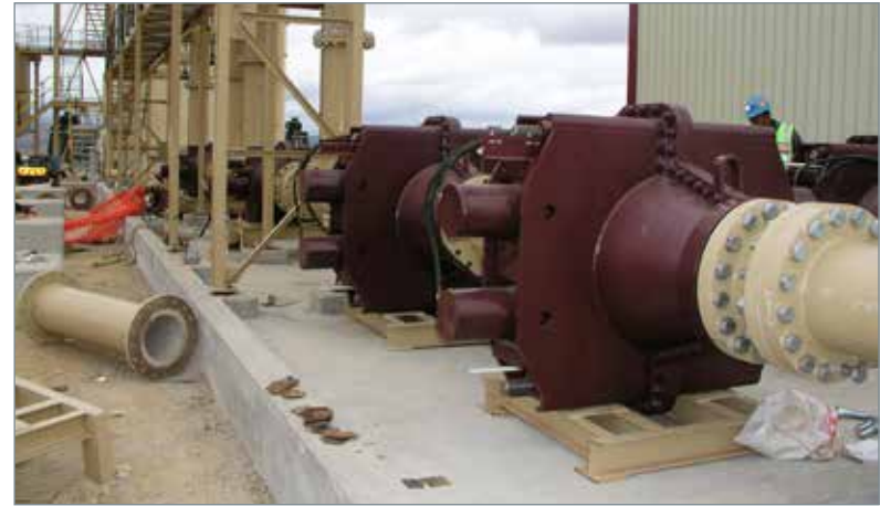
Robust Corflex pinch valves - which were designed and manufactured in South Africa by Corflex Engineering, in partnership with BMG Fluid Technology - offer a dependable solution that demonstrates sustained performance under abrasive, high-pressure conditions, with minimal maintenance. These pinch valves also boast zero operational failures since installation seven years ago.
