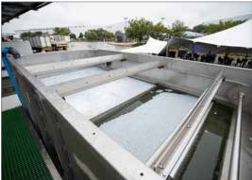
Xylem's DAF systems are increasingly being used by F&B companies to remove solids and fats at the front end of treatment.
