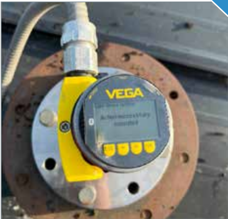
VEGAPULS 6X radar sensor delivers continuous, non-contact level measurement unaffected by dust, with no wear or clogging.
