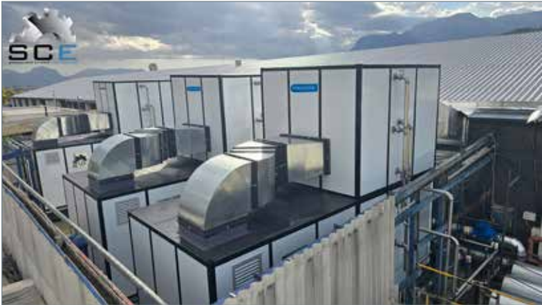
SCE's FREECOOL® air handling systems are engineered to utilise a facility's available waste heat sources as part of its conditioning process, dramatically reducing energy by up to 90%.
