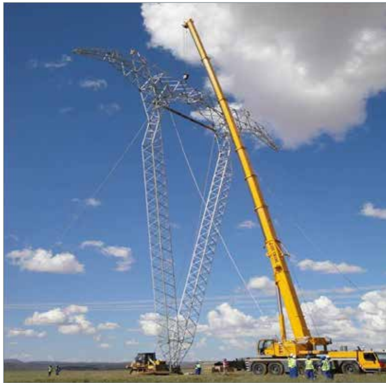
Eskom erecting transmission pylon.
