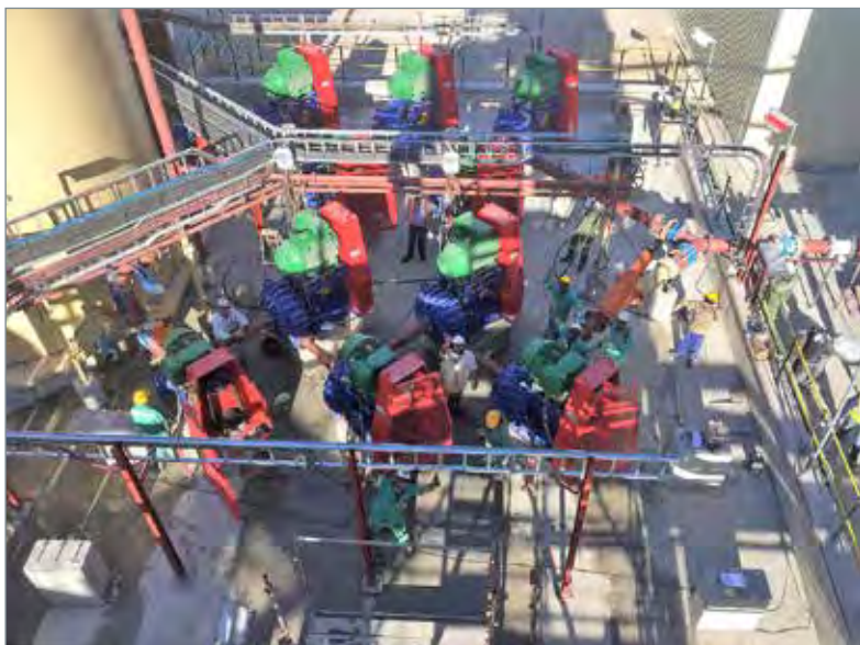
KSB Slurry pumps installation at Navachab Gold Mine, Namibia.
