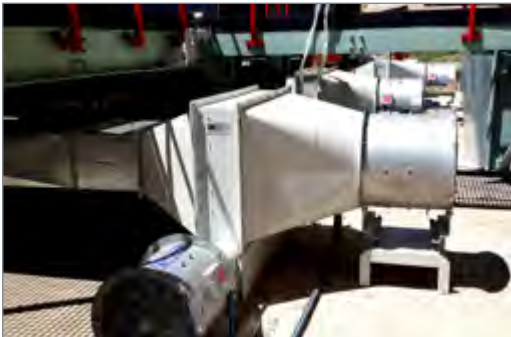
RTS Africa Engineering supplies inertial spin filters for back-channel cooling of the variable speeds (VSDs) typically used in large-scale mining or industrial projects as pictured.
