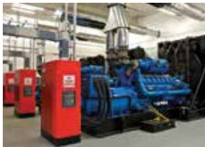
Six 2 000 kVA open type synchronising generator sets
