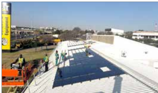
Installation of a 300kW Cat Thin Film PV solar solution by Barloworld Power for sister company Barloworld Equipment in Isando.
