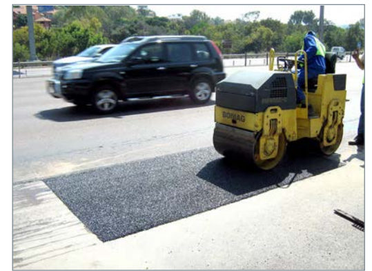
National Cold Asphalt cold mix repairs being undertaken on the N1 highway.
