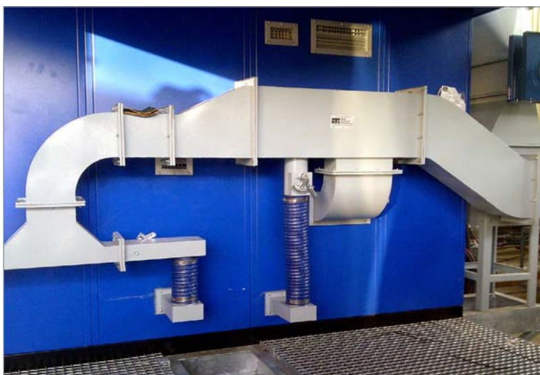
RTS Africa Engineering supplies inertial spin filters for the variable speed drive (VSD) panels typically used in large-scale mining projects such as the one pictured.
