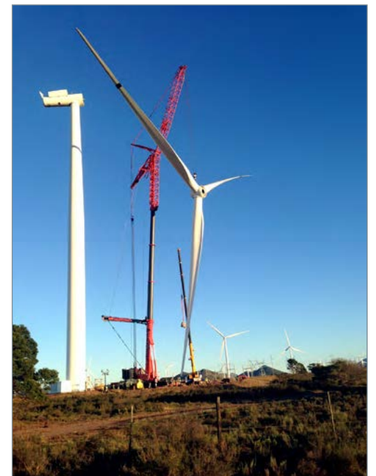
Johnson Crane Hire deploys its Liebherr LTM 1750-9.1 (750 ton) all terrain crane for a wind farm lift.
