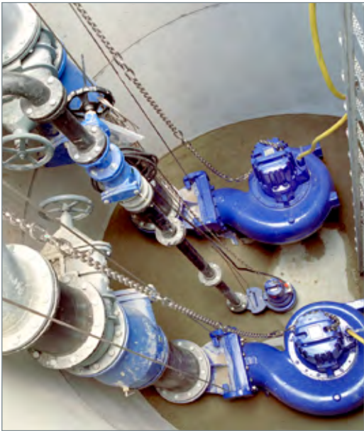
Sewatec pump installed and ready to be put into operation at a local sewage plant.
