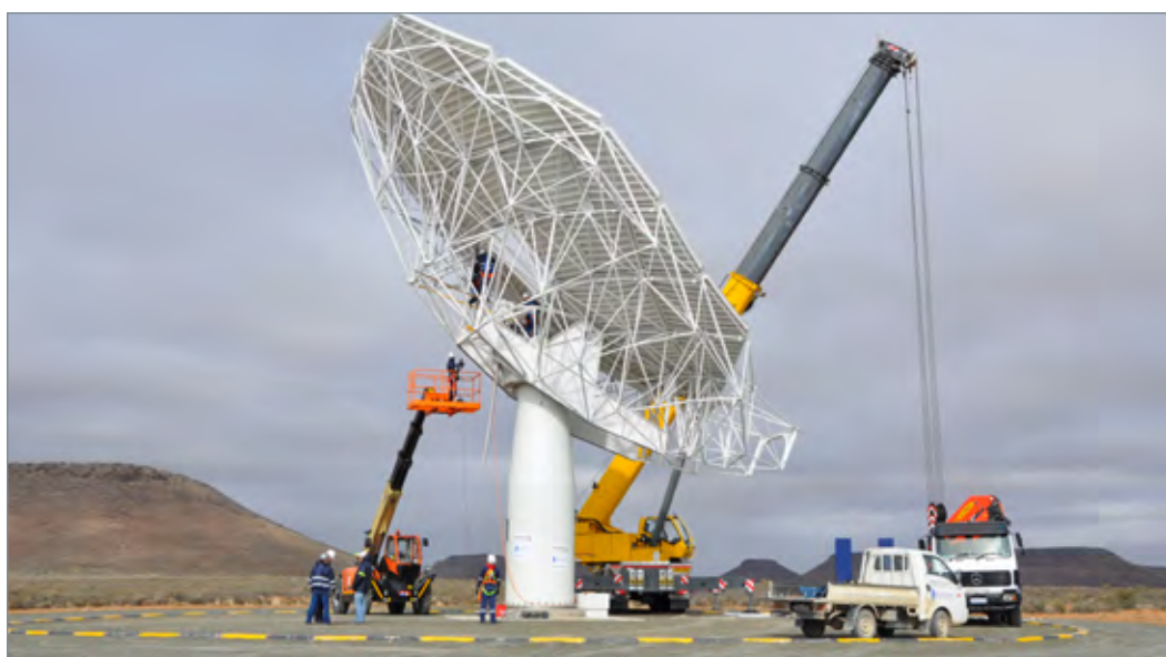
Final product; Installation of the dish onto its foundation.
