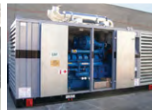
Containerised 1 250 kVA generator set
