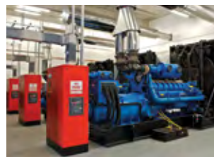
Six 2 000 kVA open type synchronising generator sets
