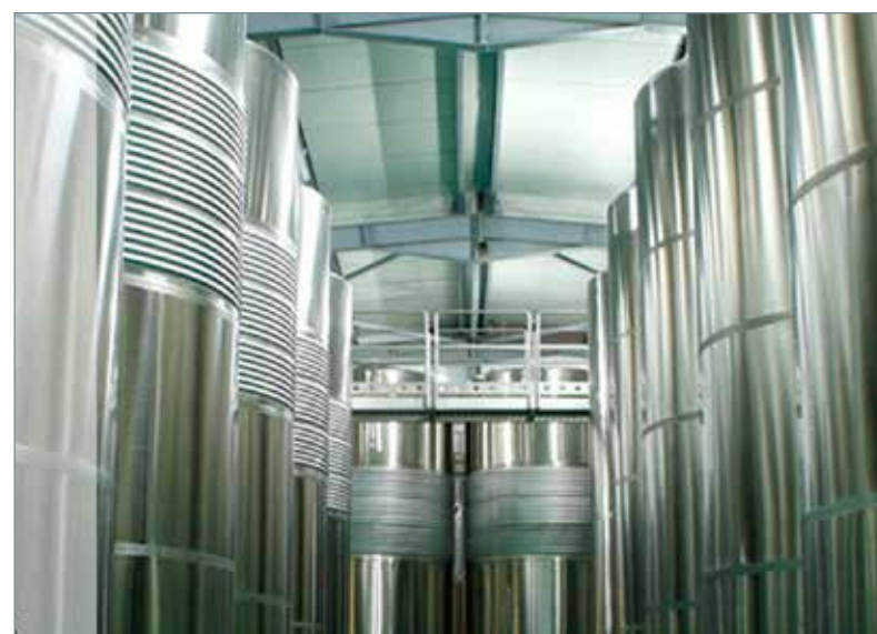
Hygienic stainless steel silos in 304/304L and 316/316L sheet and coil which is available from NDE.
