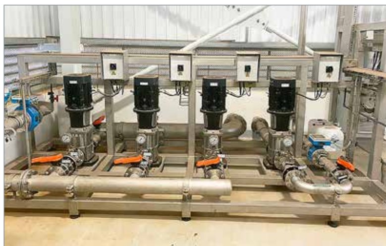
Various Grundfos 316 stainless steel multi-stage pumps pump treated water back into the brewery plant for wash and clean.
