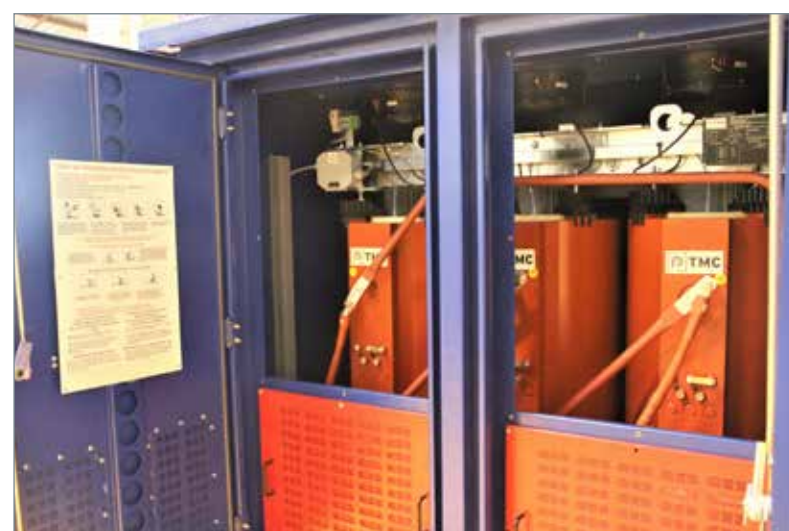
Mini substation housing built for outdoor application with 500kVA cast resin transformer.
