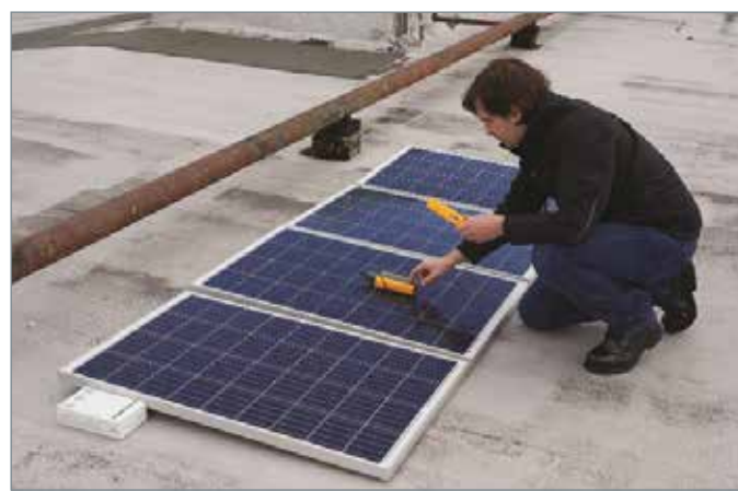
Commissioning a photovoltaic system for maximum performance.
