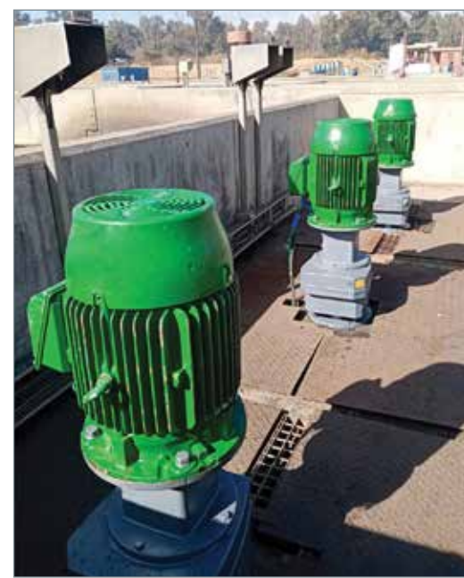
WEG IE3 motors mounted vertically on mixers for downward agitators which are used for ensuring solids entering the anoxic basin/zone do not settle at the bottom.
