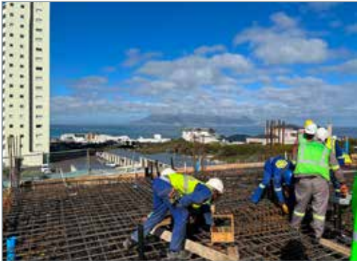
Placing of second floor slab rebar reinforcing against idyllic Table Mountain vista. Credit: Andrew Hoek.
