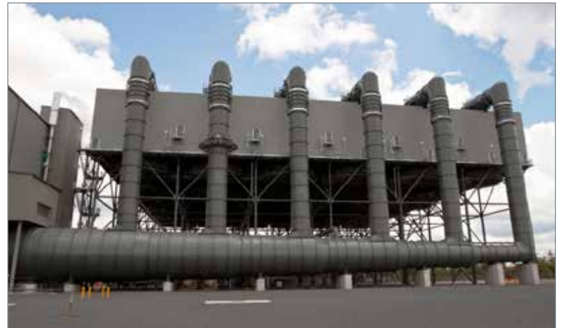
In addition to offering modular products, SEW-EURODRIVE can offer purpose built products such as the air-cooled condensers that would be used in dry cooling towers.
