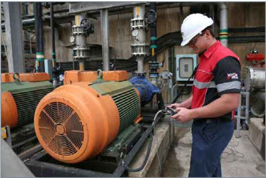
WearCheck asset reliability care (ARC) technician, Peet Peacock, performs vibration analysis testing as part of the company's wide range of condition monitoring services.
