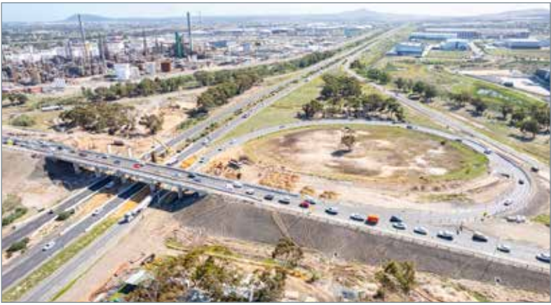
One other element of the project is the realignment of the interchange's five access ramps to suit them to the upgrade bridge structure.
