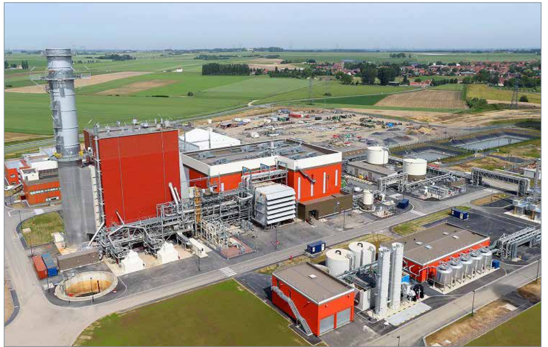
EDF Energy's combined-cycle gas turbine (CCGT) power plant at Bouchain in northern France is one of the most energy-efficient in the world, achieving an overall efficiency level of 62.22%. The plant can ramp up its output from zero to full power in only 30 minutes.
