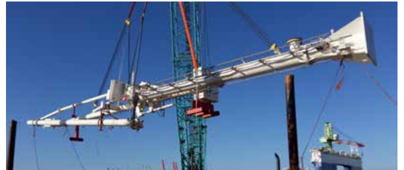
Marine loading arm installation by Soliflo
