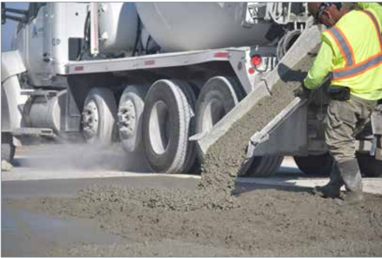
A 30 to 40 minute workability is achieved by applying the accelerator upon readymix arrival.
