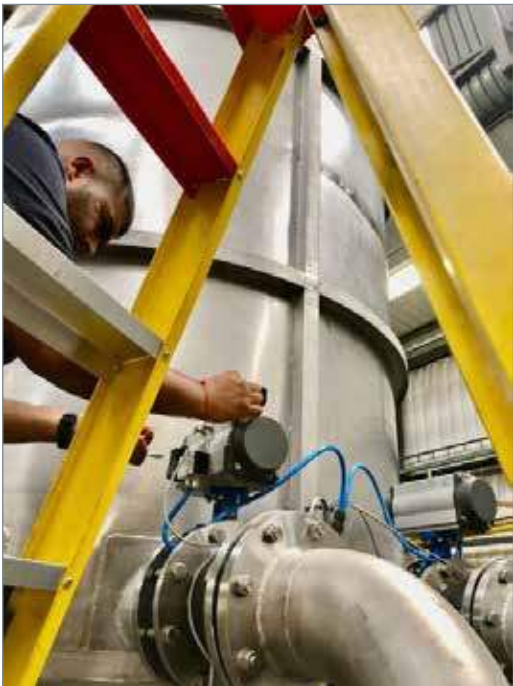
An EMVAfrica technician working on a butterfly valve to ensure the flow is regulated of abrasive slurries and to control the discharge of tailing.
