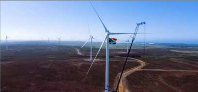
The Oyster Bay wind farm near Oyster Bay in the Kouga municipality in Eastern Cape:
